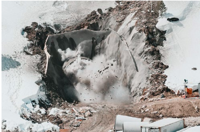
April 2021 Start of main construction work in Kühtai
