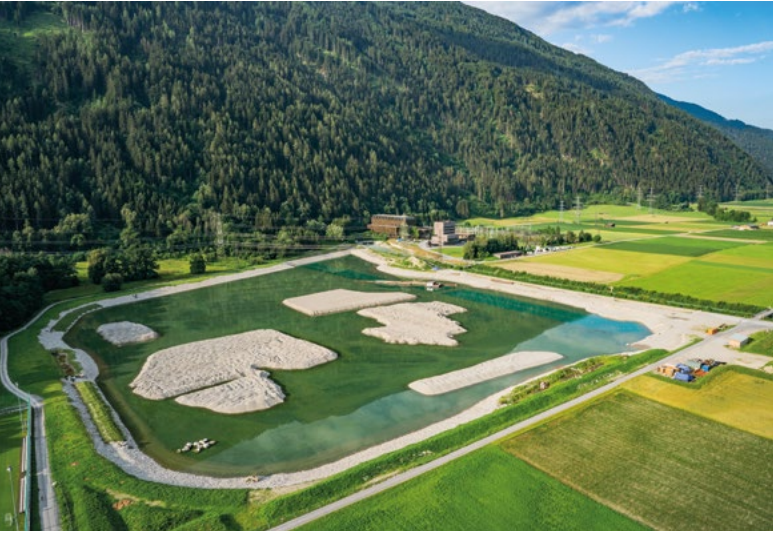
+ Europe's largest re-regulation reservoir close to Silz will significantly improve the water ecological situation along the Inn river from 2024 onwards (image shows re-regulation reservoir under construction).
