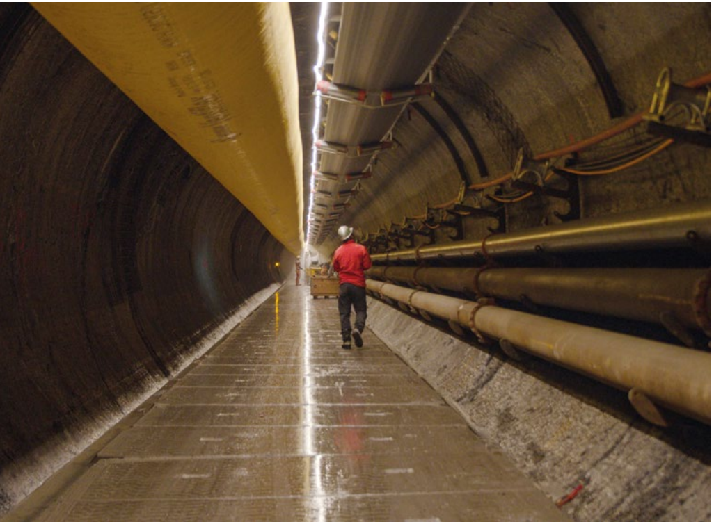
+ Inspection of the already constructed part of the diversion tunnel during the construction phase
