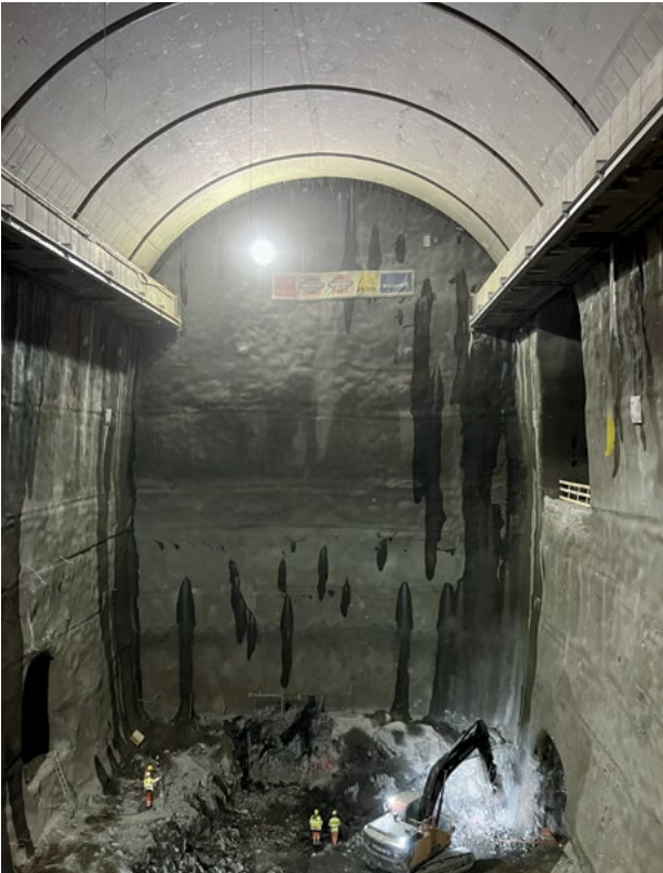
Spring 2023 The cavity blasted out of the rock for the power plant
