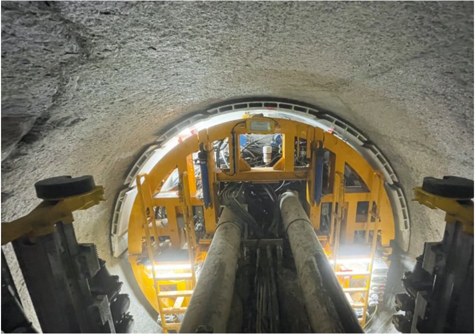
+ The diversion tunnel immediately behind the cutter head of the tunnel boring machine
