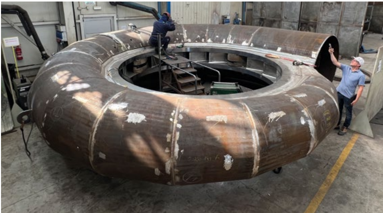
June 2023 The structural steel work on the pump turbine spirals is proceeding according to plan alongside construction
