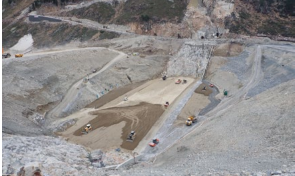
Autumn 2022 Work on the impervious core of the rockfill dam at the end of the first pouring season
