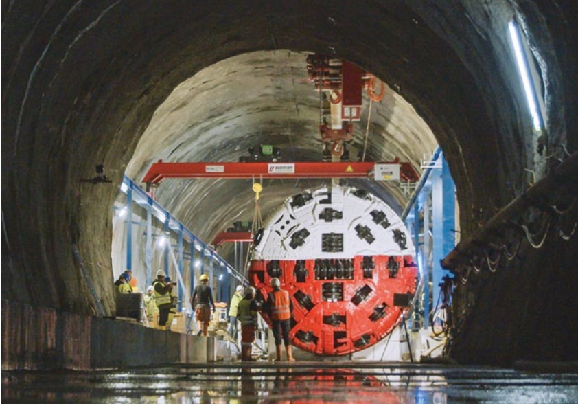
+ The ALESJA tunnel boring machine is being prepared for use
